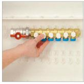
Place the assemblies inside the cabinet to find the proper location for the two connection supports (we recommend using the internal positions closer to the two ends of each manifold).
