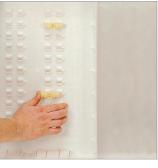
**2.** Place the R598Y003 supports over the twin dovetail-fit system and press slightly to connect them.
