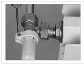
**5)** Position the clamp and tighten fully using a screwdriver.
