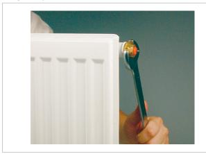
To tighten the inserts R46CF, R46CE and R46CI we suggest to use a key in size 24 mm.
