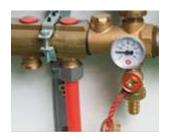
The installation must be carried out carefully to remove the air contained in the pipes. This procedure must be done manually by filling the pipes as follows:
