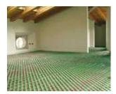
Before laying of the support layer, to make sure that during installation operations have not accidentally damaged to the pipes. You must proceed to filling loop by loop, and to vent any air pockets. After that, you can run a test with water at least twice the working pressure and not less than 6 bar.
