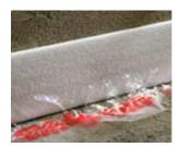
The perimeter wall insulation band must be placed along the walls and along any other component that penetrates into the base foundation (for example columns). It is an insulating band that connects the base with the finished floor. This in turn allows small movements of the top layer (few millimeters). The band should be secured to the ground so as to avoid movement during the casting of concrete. The upper part of the perimeter band will be cut only when the entire floor covering is completed.
